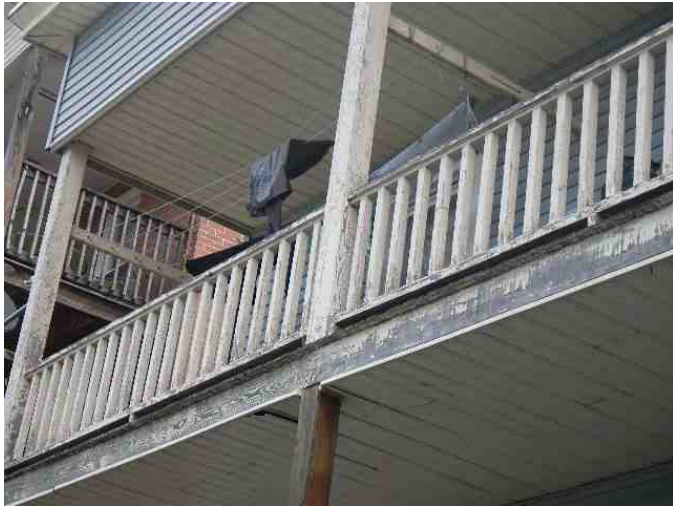
Loose paint of porch
